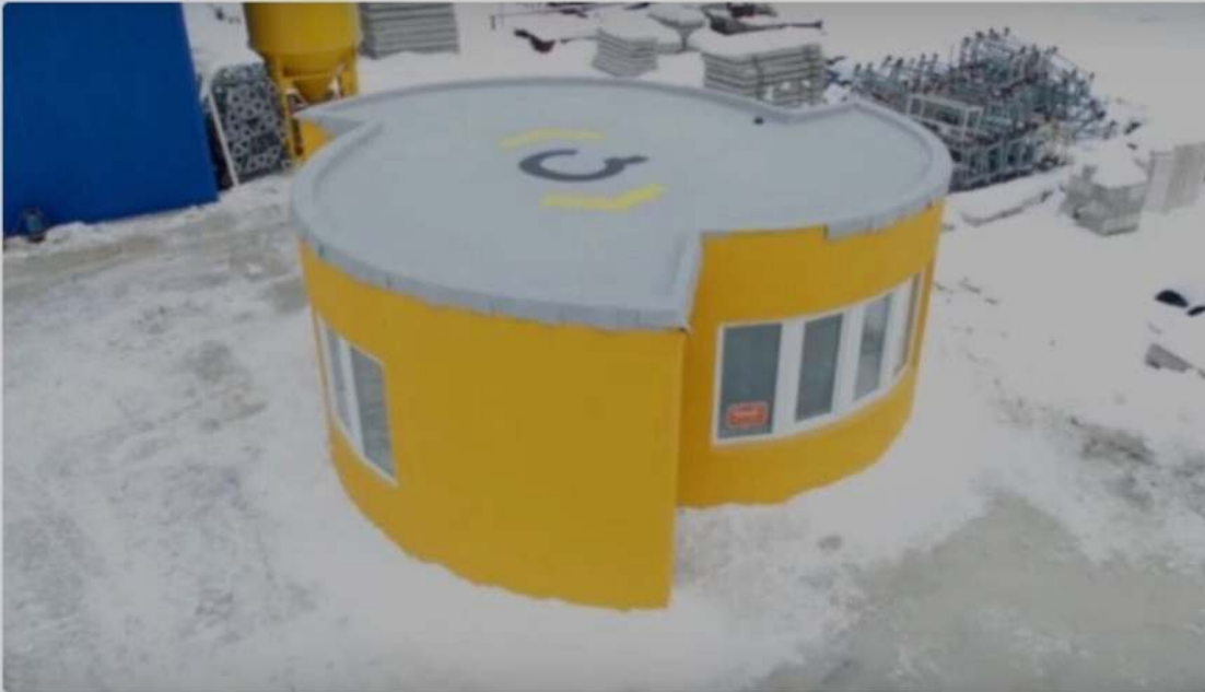
Apis Cor built this magnificent 3D printed house in just 24 hours!
